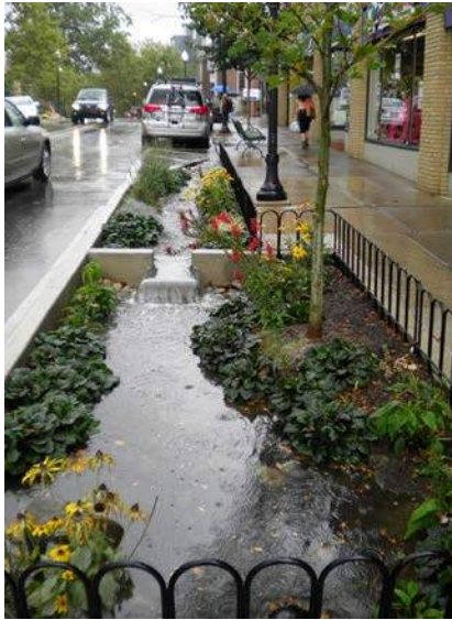
Photograph 2. One of two rain garden retrofit projects installed at the corner of Allen Street and Beaver Ave in the Borough of State College
