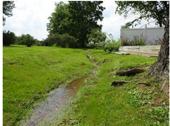
Photograph 2. Sediment deposition in channel
